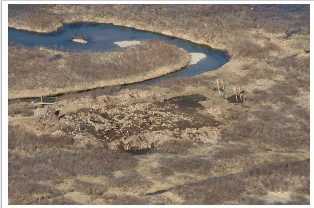
Pic. 1. Overview of the excavation area.
