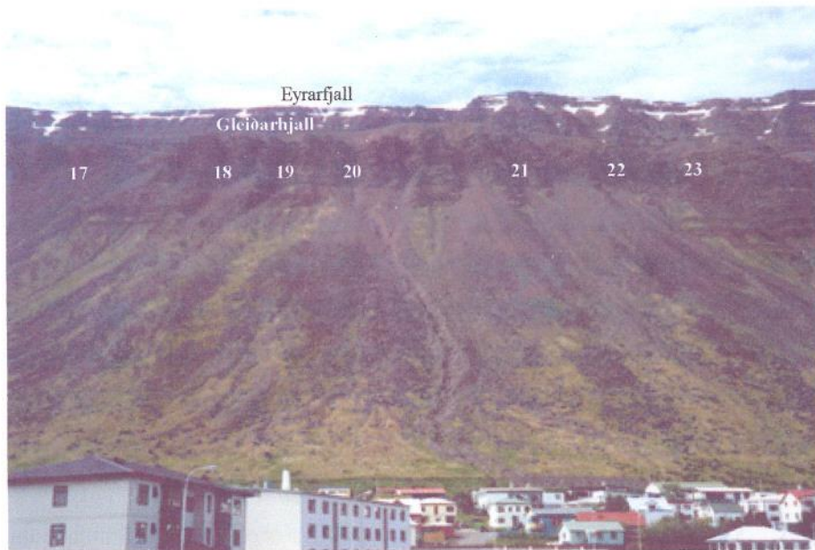
Figure 10: Overview of the outer part of the Eyrarhlíð slope. The picture is taken towards northwest.
